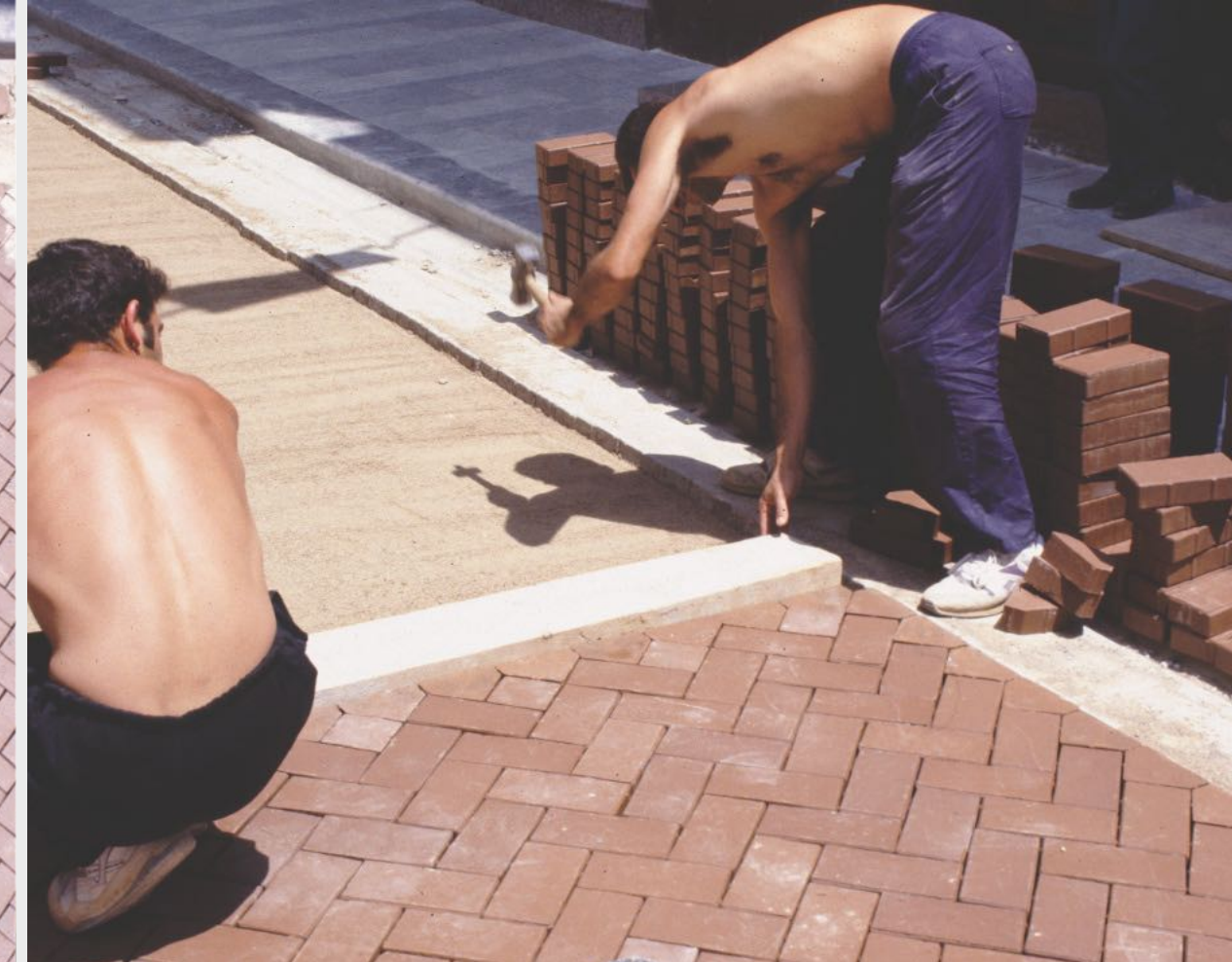
Aligning pavers
