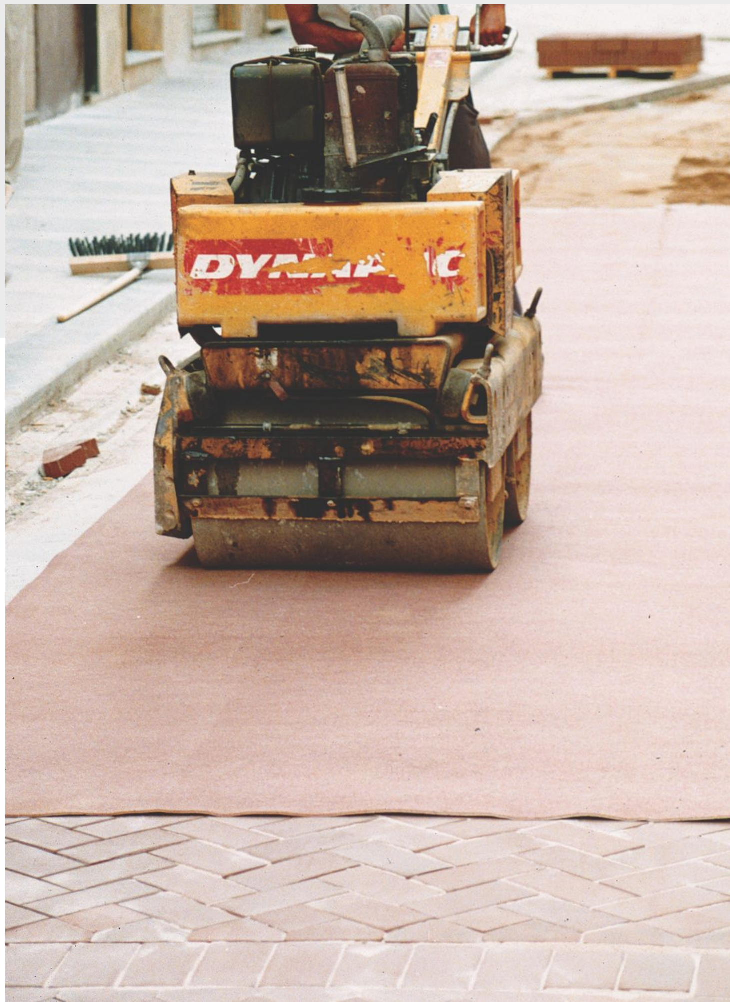
Compacting pavers. Use vibrators with rubber bases, or spread out a blanket as shown in the photo to avoid chipping.
