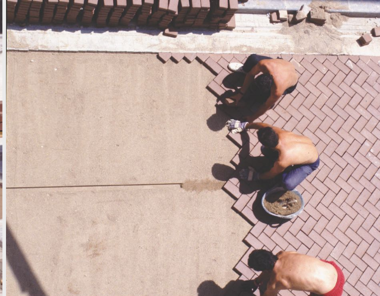
The laying of pavers
