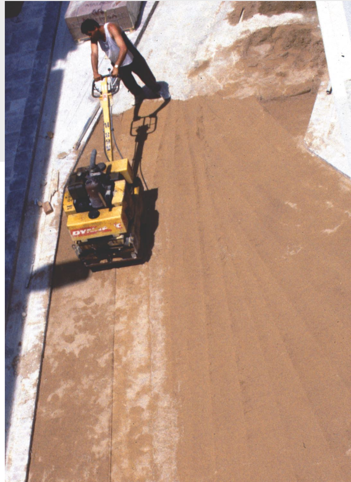
Levelling and sand compaction
