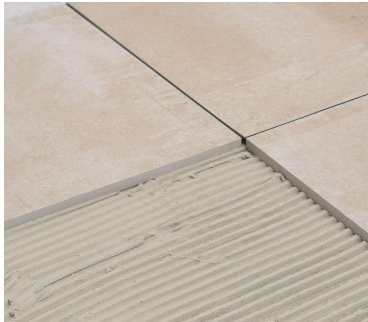
**EN** The conventional tile-laying method can be used for all outdoor areas, on open or covered terraces, parking areas, entrance or exit ramps, poolside and spa areas etc. This method is the most resistant to heavy loads.
